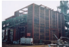
Installation of large shredder
