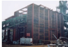
Installation of large shredder
