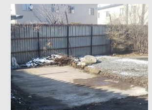
After garage removal
