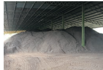
Mine Biomass Synergies PKS Stockyard
